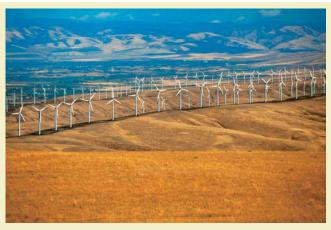
This State Line Wind Project along the Oregon-Washington border uses approximately 399 wind turbines to create enough electricity to power some 70,000 households.
